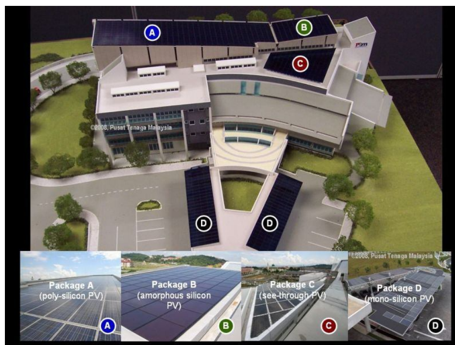
Figure 8. Four types of solar panel and their locations on the GEO building [20]
